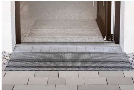
Figure 4.6 Channel drain at entrance door
